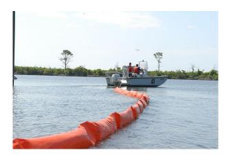
Crews also used long pieces of plastic called booms to contain the oil on the surface. Booms were used to trap oil and prevent it from washing up on shore. Workers placed millions of feet of booms along the coasts of the Gulf of Mexico.
